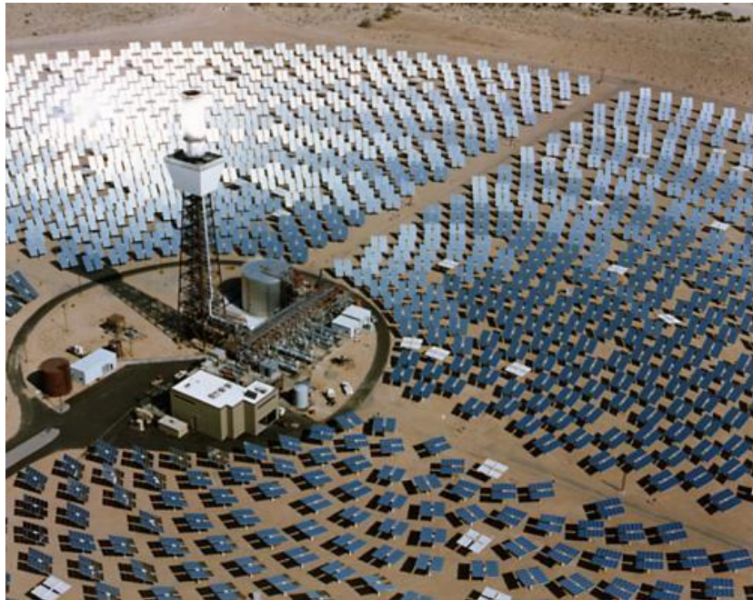
Figure 2. “Solar Two”, a solar power plant in California. (INFORSE 2006)
